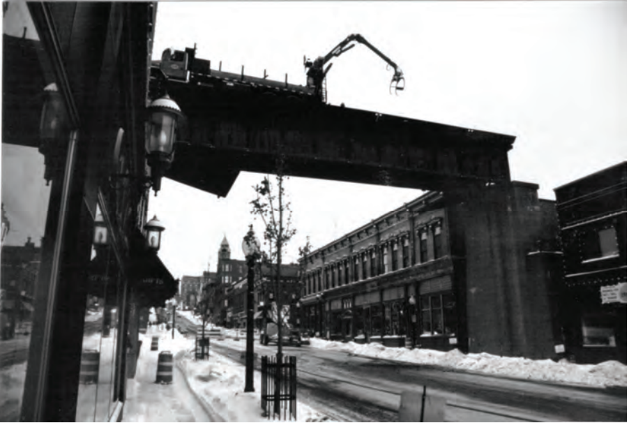
Railroad trestle removal in downtown Marquette (1999-2000) Photo Credit: Sonny Longtine
